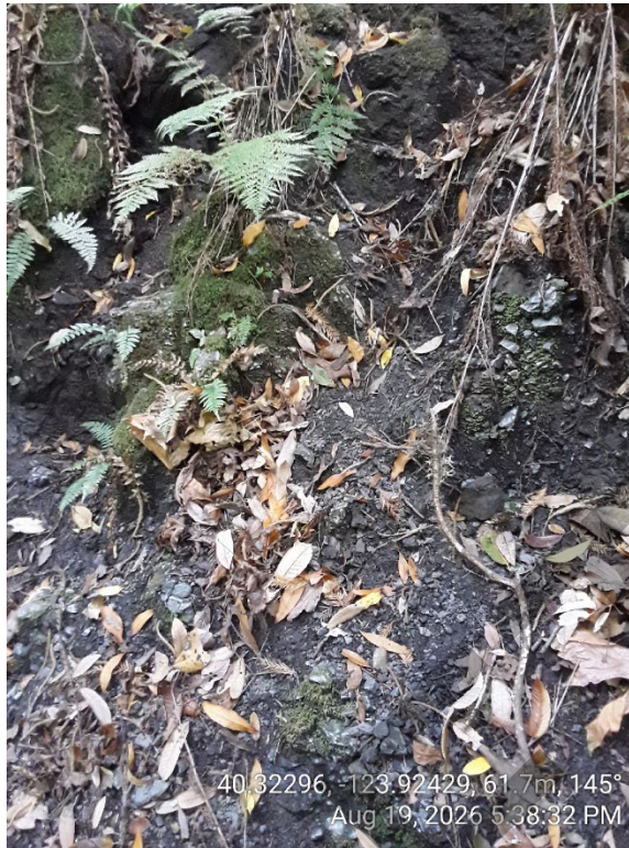
Location 5- Bedrock Exposed in Channel Bank w/Seep
